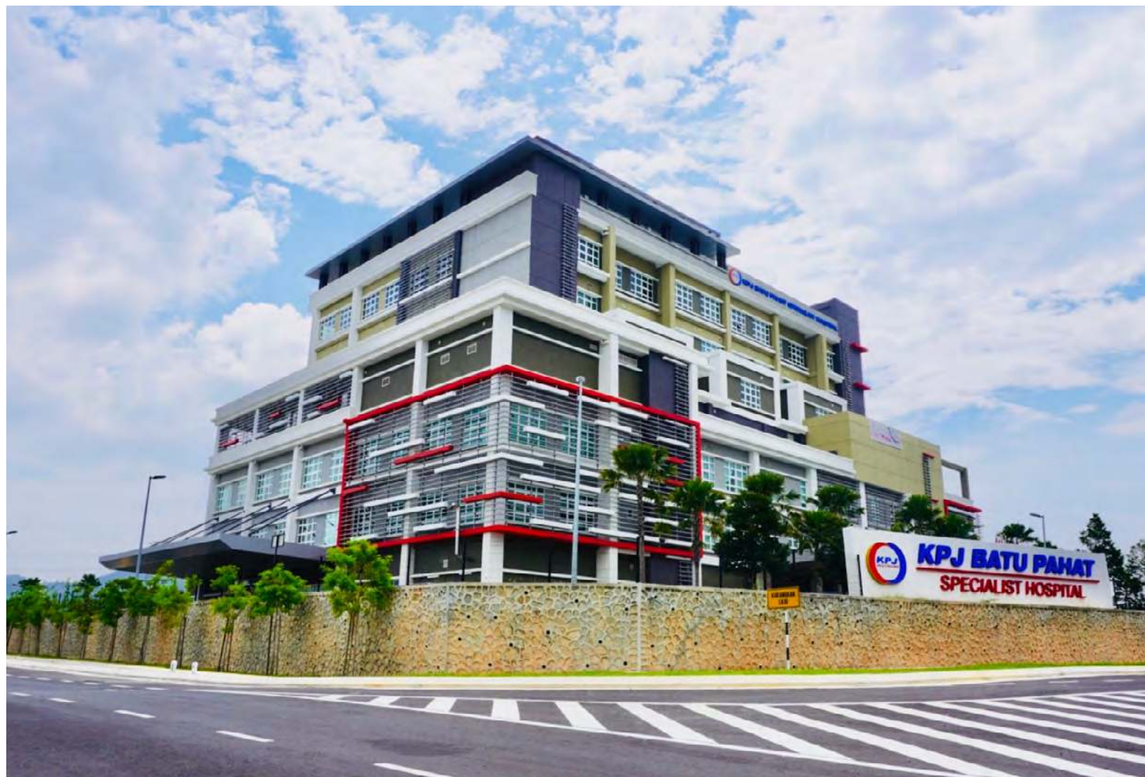
KPJ Batu Pahat Specialist Hospital, the 23 rd asset owned by Al-Aqar.
